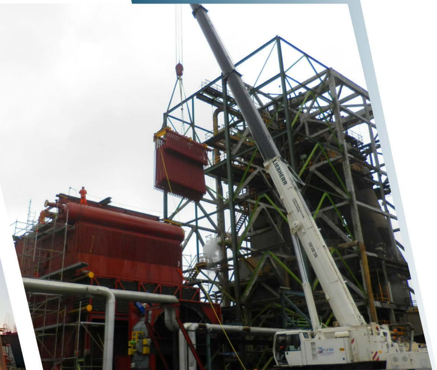
Boiler Substitution
